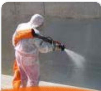
Mobile coating on-site
